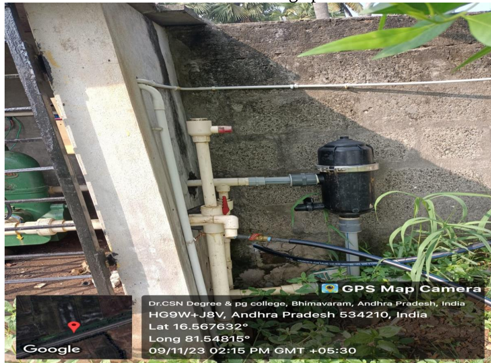
Bore well in our college premises
